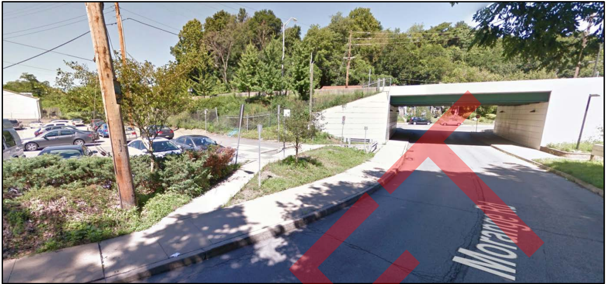
Figure 4-2: Culvert at the Morange Road Flooding Location (Multiple Inlets Near Underpass)
