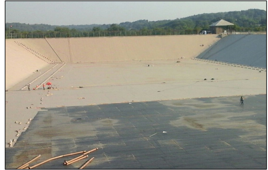
Lanpher Reservoir (Completed)
