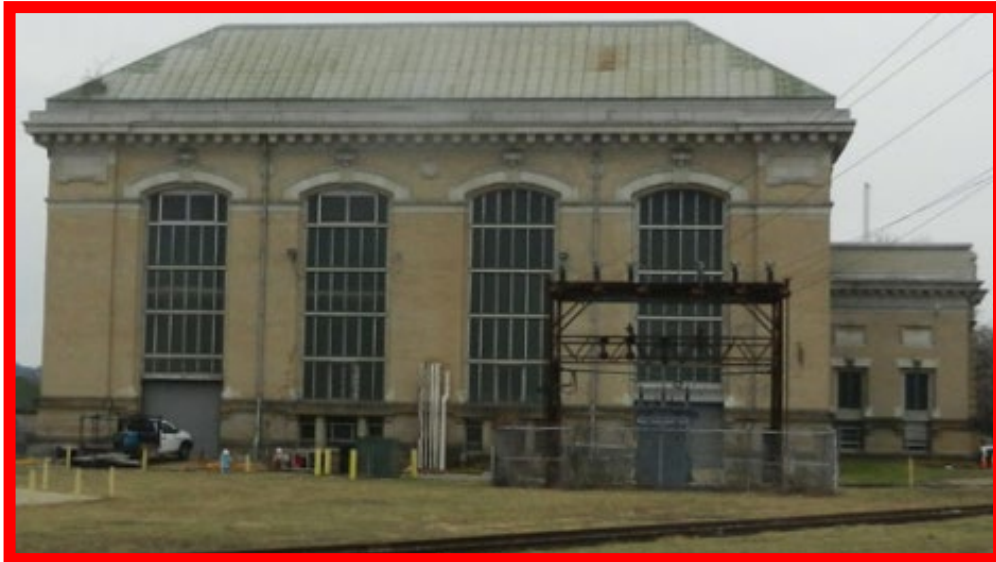
Aspinwall Pump Station
