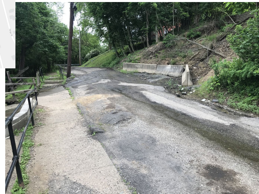
Remediation of landslide and seep impacts on road and drainage
