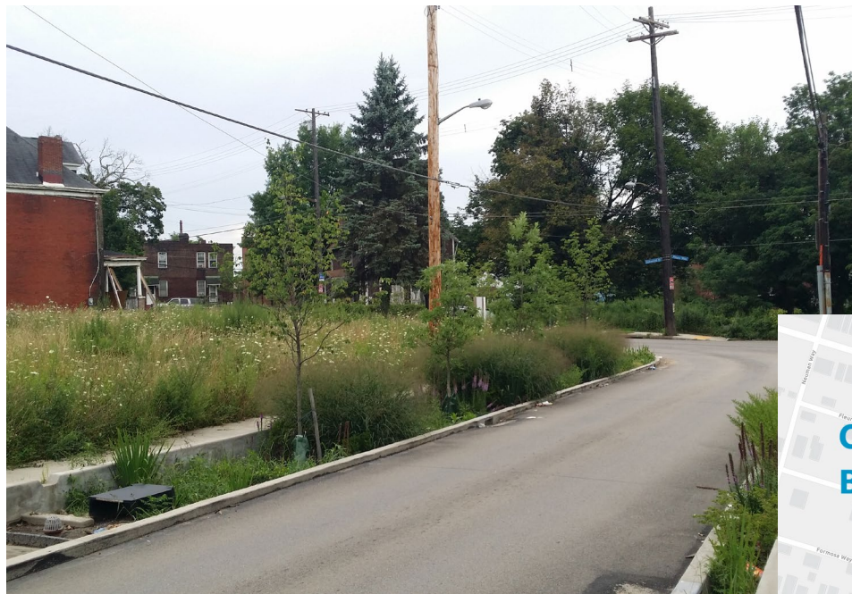
Renovation and repair of green stormwater infrastructure (GSI)
