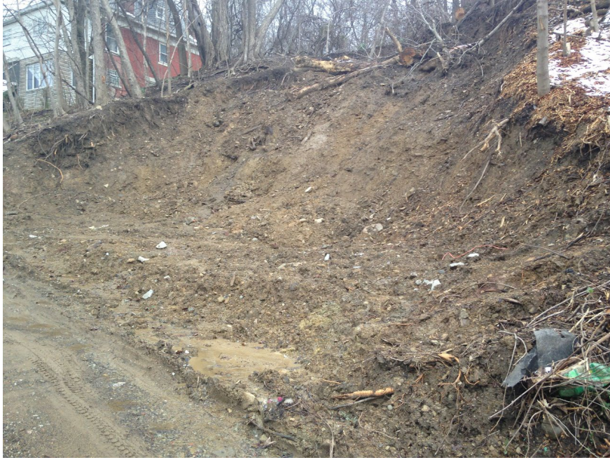
2018 Landslide on Haverhill St.
