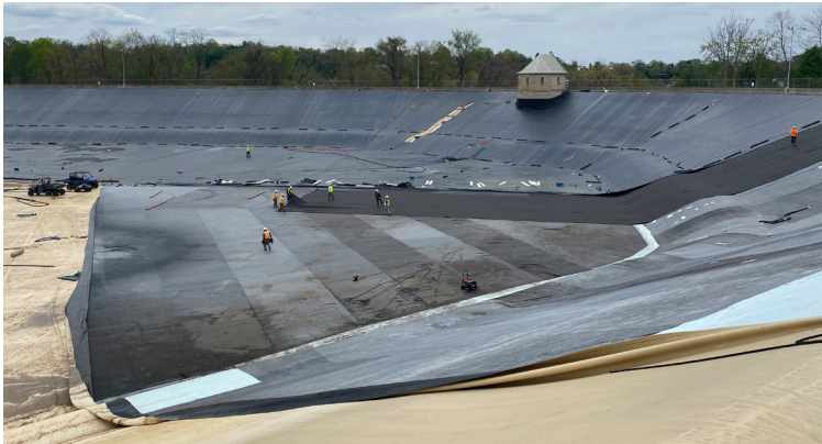
Crews begin to install new liner on the Highland II Reservoir.
