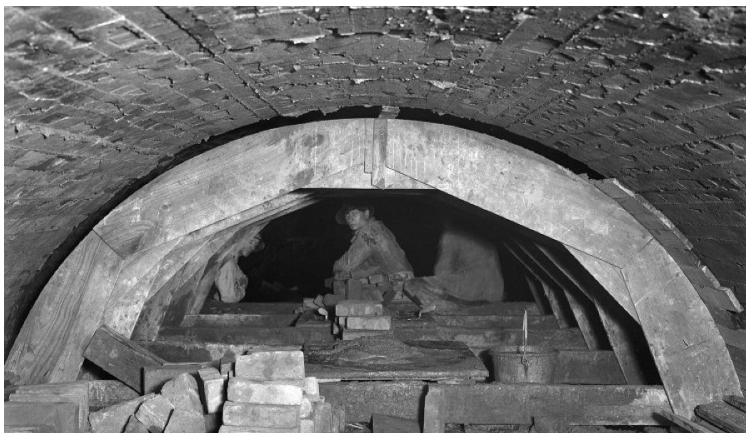
Historic image of PWSA sewer being constructed
