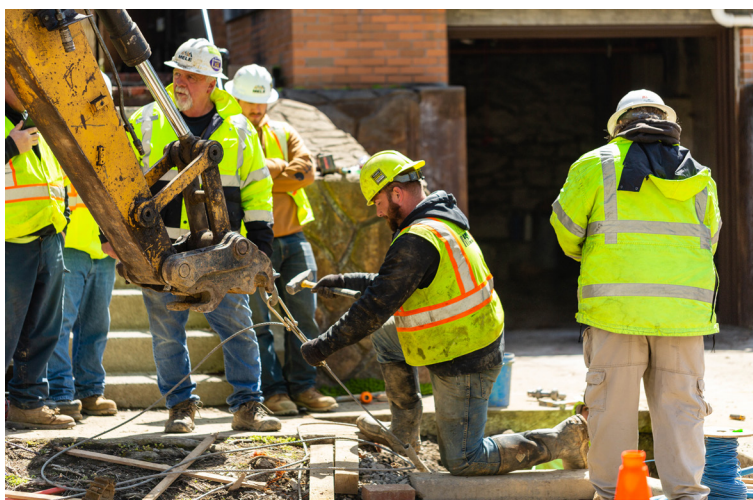
PWSA contractor crews coordinate a successful lead service line replacement.
