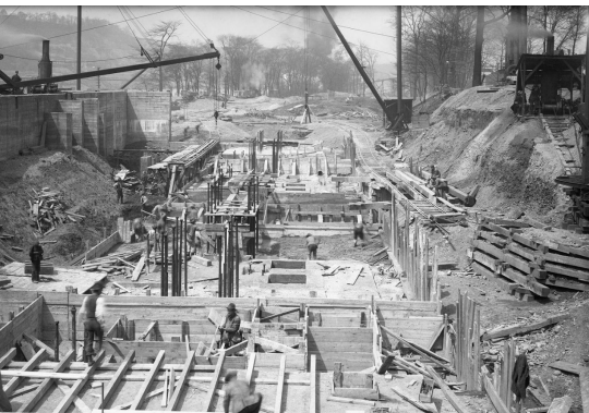
Pittsburgh's first filtration plant construction in 1906.
