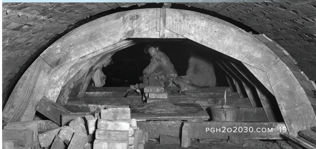
Historic 1914 photo of sewer construction in Pittsburgh
