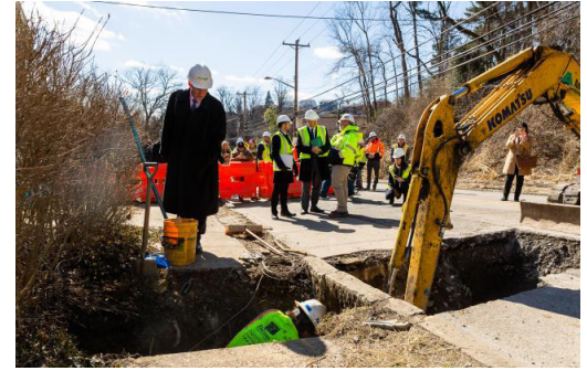
Lead service line replacement work being performed on Hazelwood Ave.
